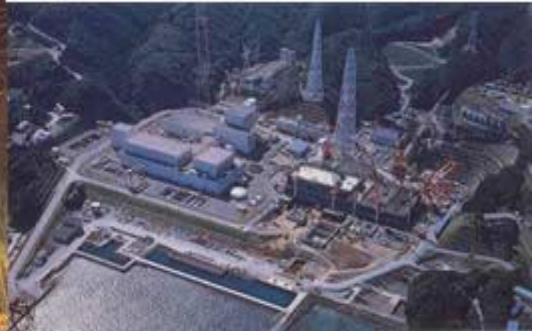
▲ Nuclear power station
