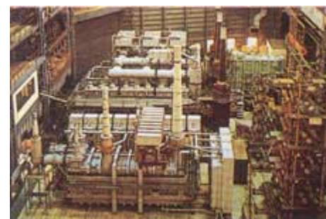
Fig.18 Transformer Final Testing
