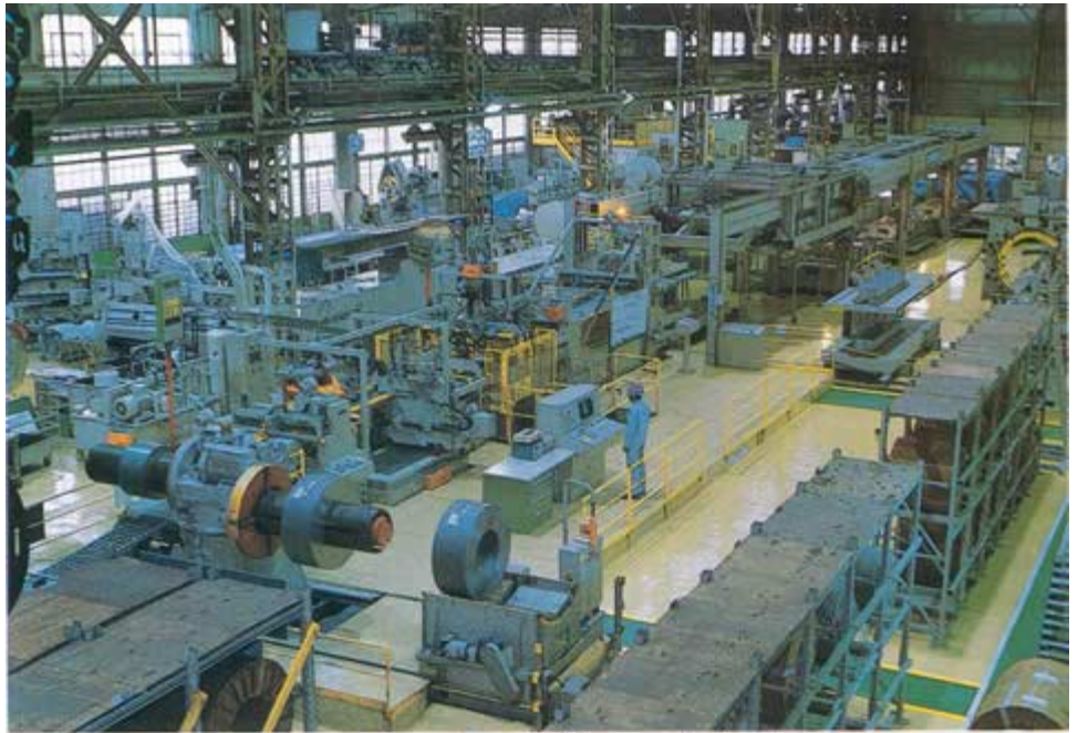
Fig.6 Computer-controlled Core Lamination Line
