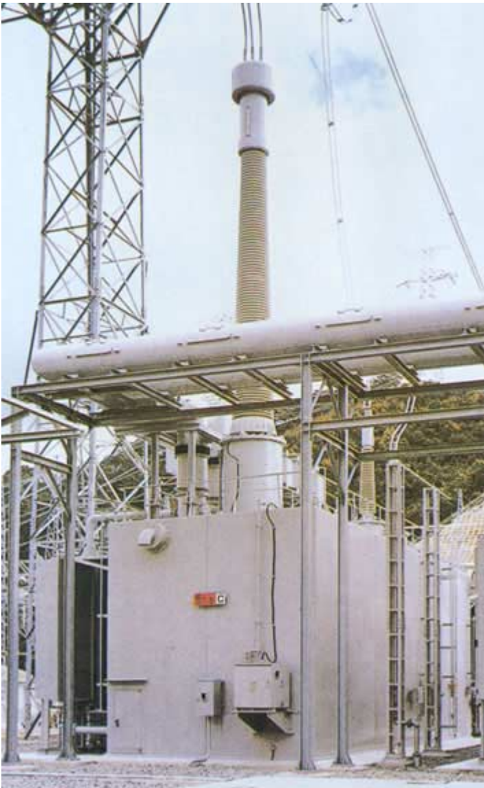
Fig.44 Steel-panel Noise Enclosure
