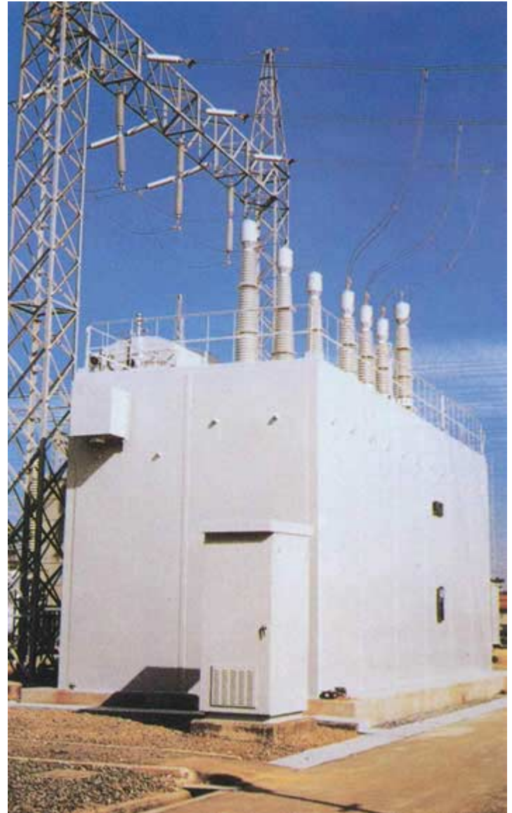
Fig.45 Concrete-panel Noise enclosure
