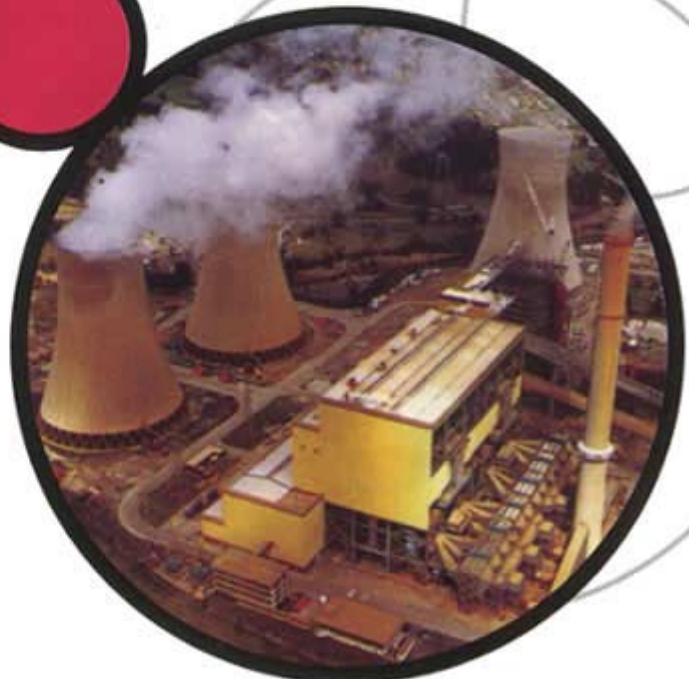
YALLOURN POWER STATION
