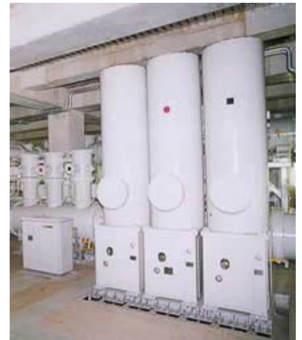
1 break GCB for 550 kV GIS in underground substation
