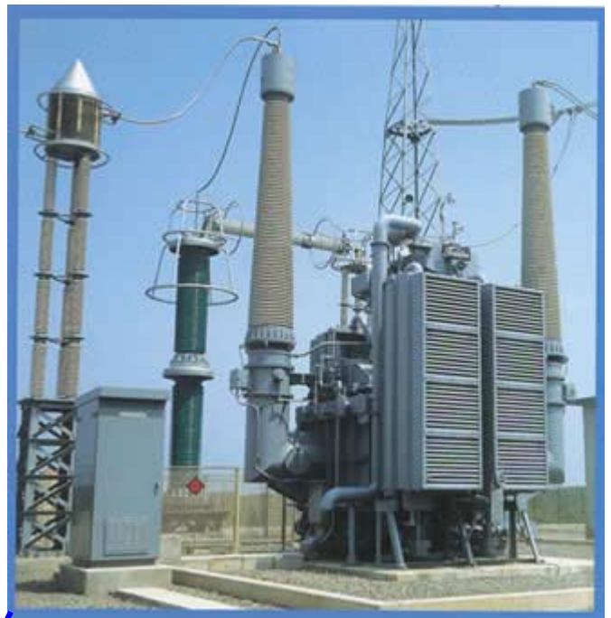
The picture shows a DC smoothing reactor and a DC surge arrester for an HVDC link.
