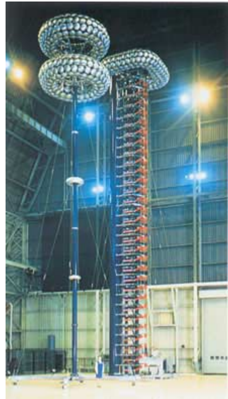
6000kV, 600kJ impulse generator in the Ultra High Voltage Laboratory.
