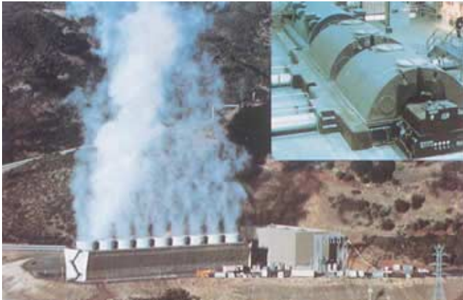
Geysers Geothermal Power Plant Pacific Gas & Electric Co., USA 6x55MW, 2x110MW, 1x114MW 4x124MW
