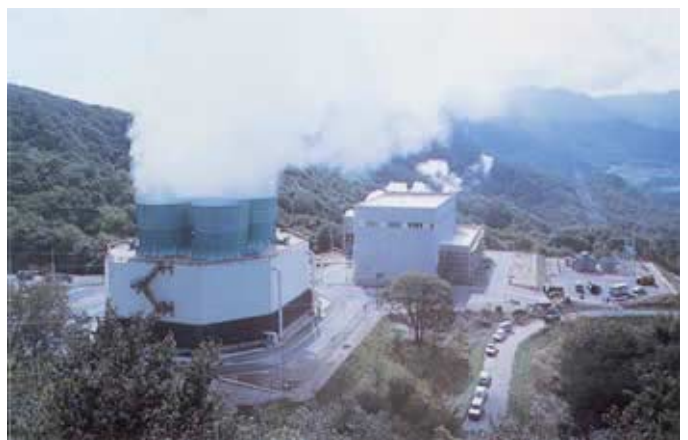
Mori Geothermal Power Plant Hokkaido Electric Power Corp., Japan 1 x 50MW
