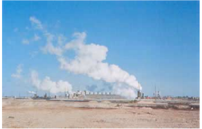
Cerro Prieto Geothermal Power Plant Commission Federal de Electricidad, Mexico 4x37.5MW, 4x110MW
