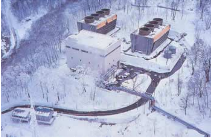
Kakkonda Geothermal Power Plant Tohoku Electric Power Corp., Japan 1 x 50MW
