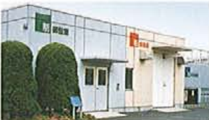
食堂排水処理施設 Restaurant waste water treatment plant
