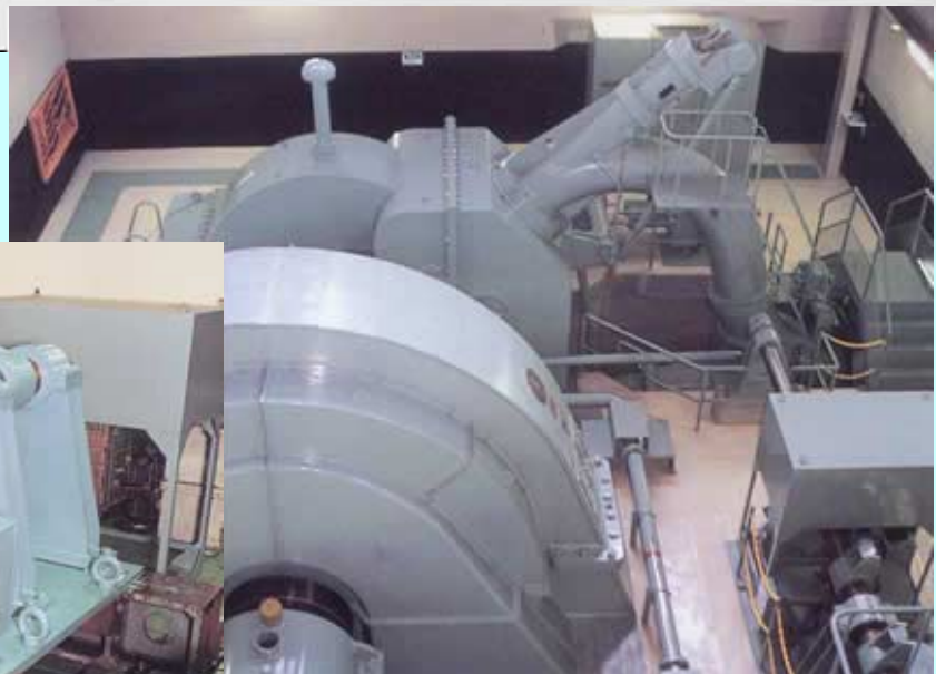
6310KW HORIZONTAL PELTON TURBINE
